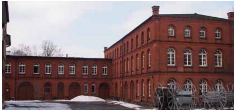
Abb. 2: Ziegelsteinbau der Stadtwerke Hof. Fig. 2: Brick stone building of public utility company Hof.
