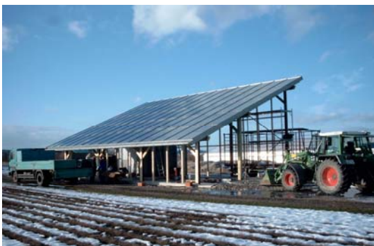
Abb.2.4.9: Solar Drying Plant Krimmer-Pulling
