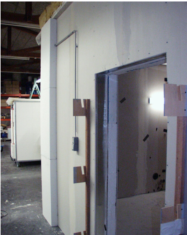
Fig. 3: External view of the test room. Numerous temperature sensors are installed inside the room to record the room climate.
